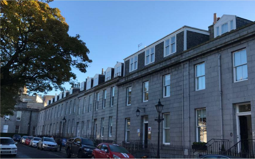
Example of a poorly designed roof extension – The modern box dormer is too large, thus it dominates the roof slope on an otherwise traditional terrace.
